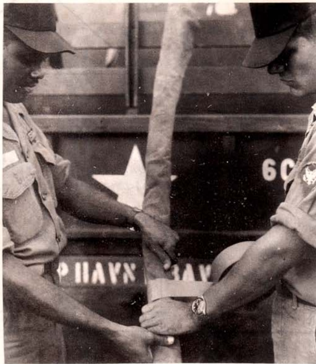
Figure 10b Final Taping of Canvas Wrapping
